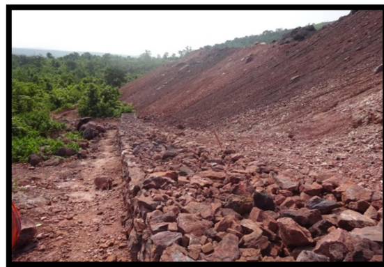
Retaining wall provided at the toe end of the dump
