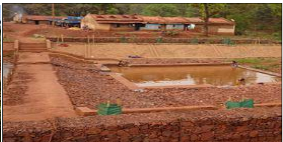
Photo Showing varies Nallah protection measures under taken out side ML
