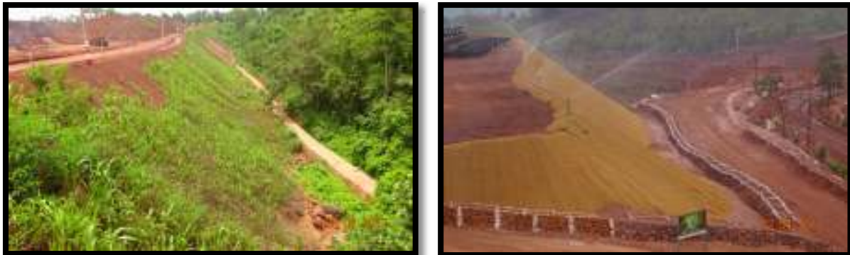
Retaining wall provided at the toe end of the dump
