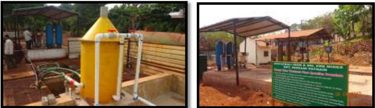
PHOTOS SHOWING STP TECHNICAL STRUCTURE & EXISTING PLANT
