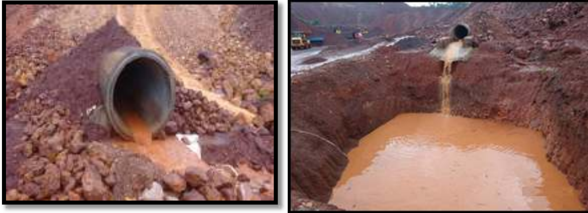
Photo showing OB & sub grade dumps are provided with retention wall and other Mitigative measures.
