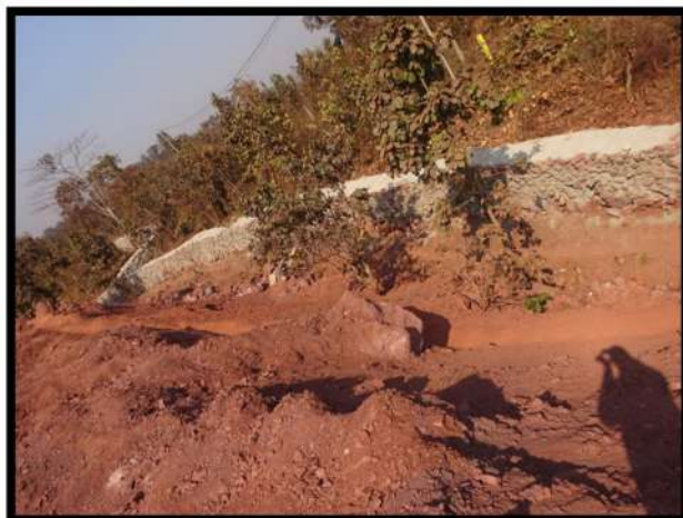
Retaining wall provided at the toe end of the dump
