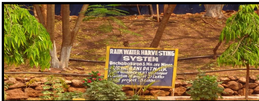
PHOTO SHOWING ROOF RAIN WATER HARVESTING SYSTEMS EMPLOYEE’S CAMP
