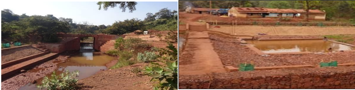
Photo Showing varies Nallah protection measures under taken out side ML
