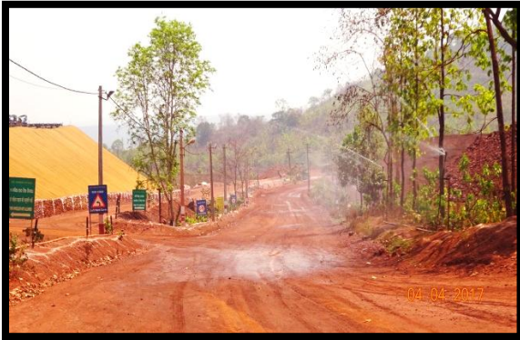
Photos showing automatic fixed sprinkler installed at mines permanent Haul road
