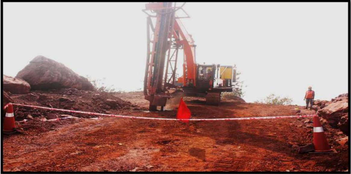
Photo Showing Excavated Mounted Drilling Machine equipped with dust extractor & wet drilling mechanism
