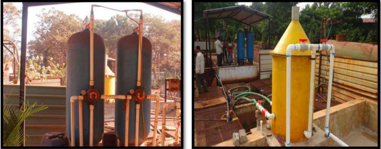
PHOTOS SHOWING STP EXISTING PLANT
