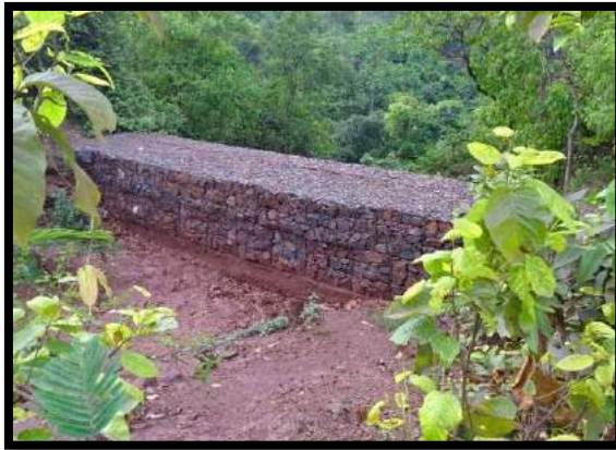
Photo showing check dams & Check weirs implementation within ML
