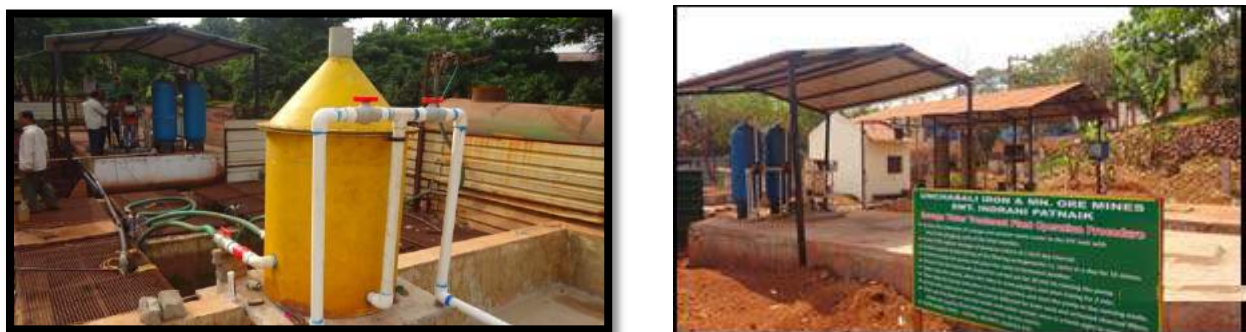
PHOTOS SHOWING STP TECHNICAL STRUCTURE & EXISTING PLANT
