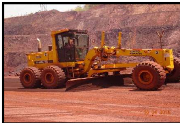
Photo showing motor grader under use for road maintenance
