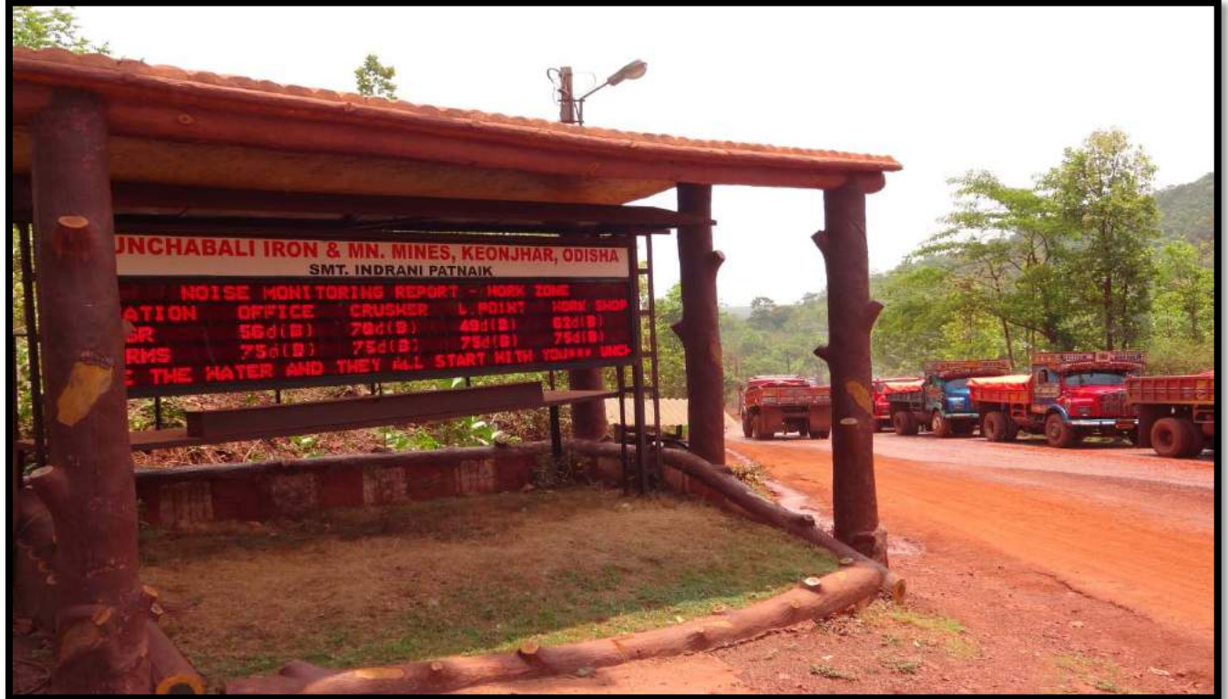
Photo Showing Electronic Display board placed in the mines entrance gate to display the Environmental parameters
