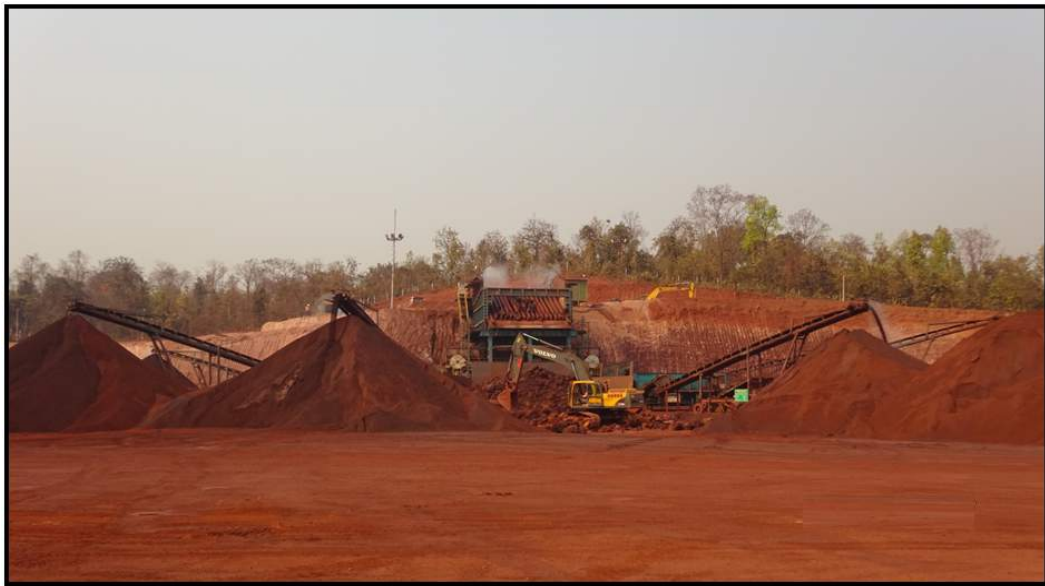
Photos showing dry fog implementations is various crusher & screen plants
