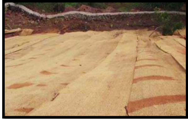
Retaining wall provided at the toe end of the dump
