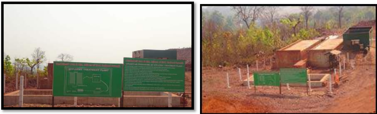
PHOTO SHOWING ETP PLANT PROVIDED IN WORK SHOP SERVICE CENTER
