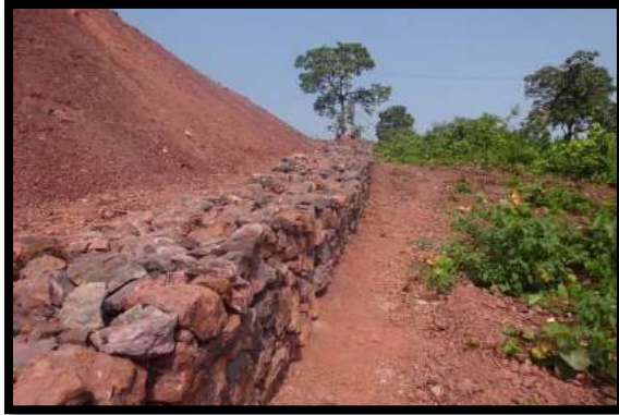
Retaining wall provided at the toe end of the dump
