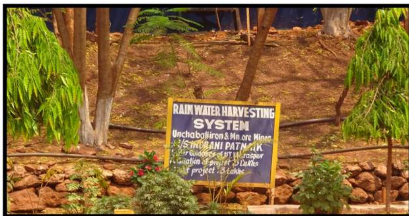
PHOTO SHOWING ROOF RAIN WATER HARVESTING SYSTEMS EMPLOYEE’S CAMP
