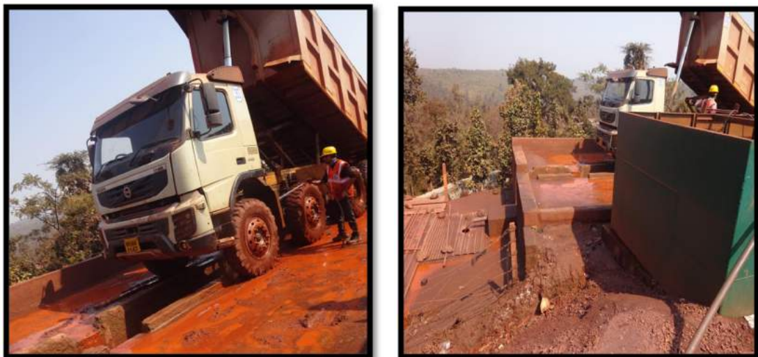
PHOTO SHOWING ETP PLANT PROVIDED IN WORK SHOP SERVICE CENTER
