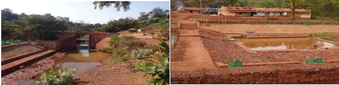
Photo Showing varies Nallah protection measures under taken out side ML
