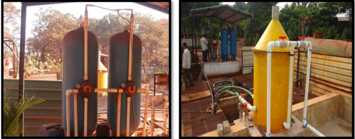
PHOTOS SHOWING STP EXISTING PLANT
