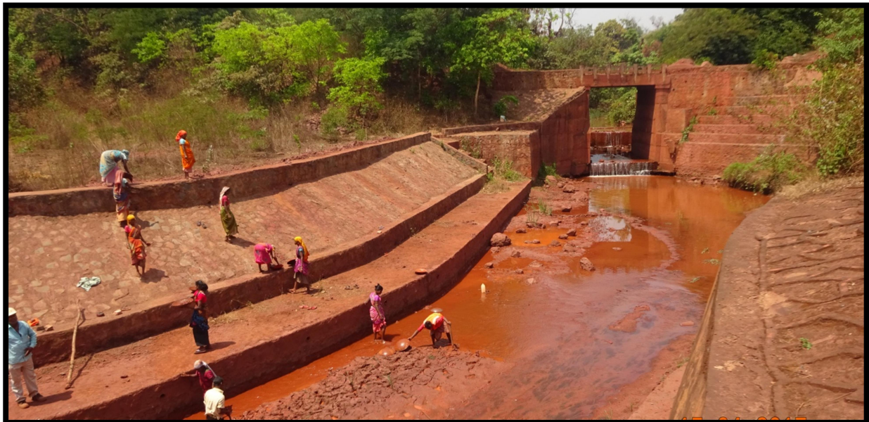
PHOTO SHOWING THE DESILTATION WORK FOR NALLAH PROTECTION MEASURES
