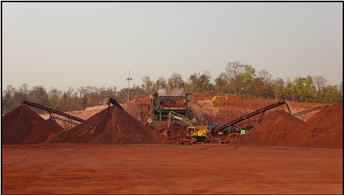
PHOTO SHOWING THE DRY FOG SYSTEM FOR THE DUST SUPPRESSION
