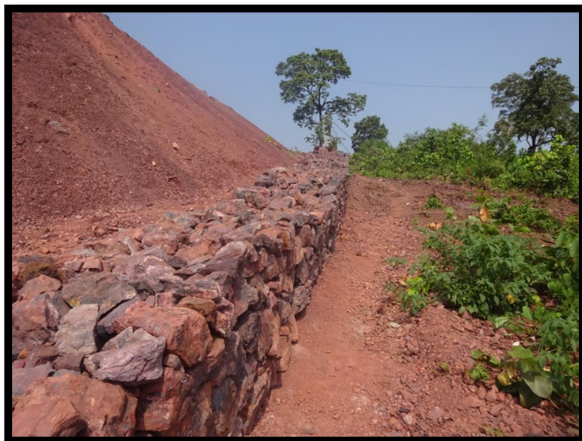
PHOTO SHOWING THE WASTE MANAGEMENT WITH COIR MATING AND RETAINING WALL
