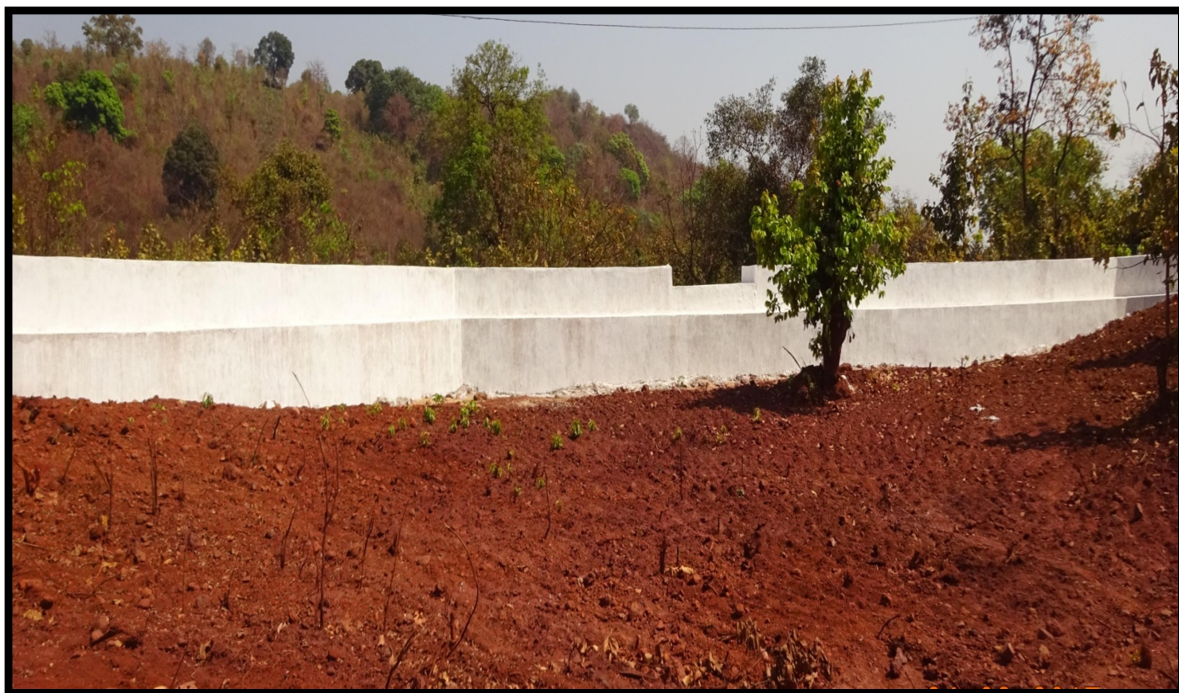
PHOTO SHOWING THE CHECKDAM CUM SETTLING POND FOR THE SURFACE RUNOFF
