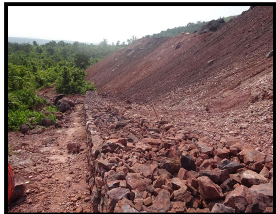
PHOTO SHOWING THE WASTE MANAGEMENT WITH COIR MATING AND RETAINING WALL
