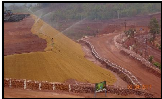
Retaining wall provided at the toe end of the dump
