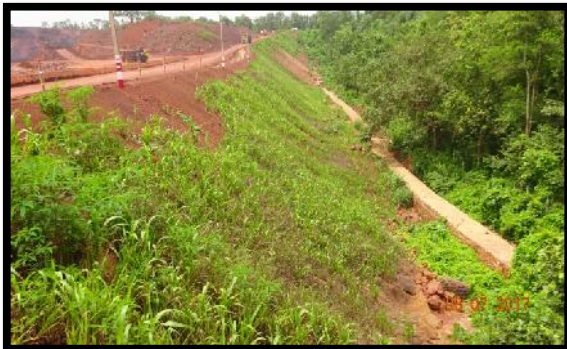
Retaining wall provided at the toe end of the dump
