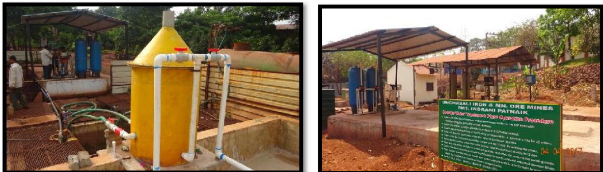
PHOTOS SHOWING STP TECHNICAL STRUCTURE & EXISTING PLANT
