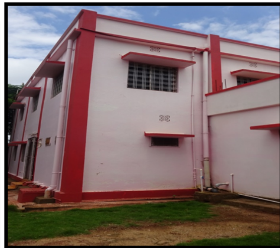
PHOTO SHOWING ROOF RAIN WATER HARVESTING SYSTEMS AT MINES EMPLOYEE'S CAMP & UNCHABALI DISPENSARY
