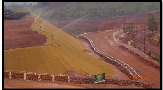
Retaining wall provided at the toe end of the dump
