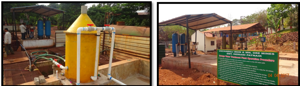
PHOTOS SHOWING STP TECHNICAL STRUCTURE & EXISTING PLANT
